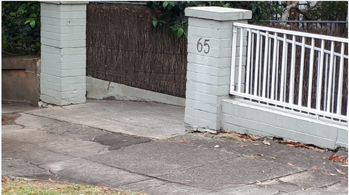
PHOTO 1 – CRACKED DRIVEWAY
